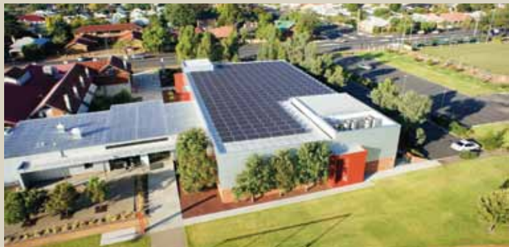
Dubbo Western Plains Cultural Centre solar panels
