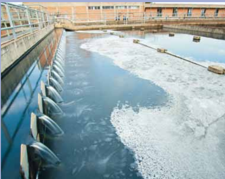
Bathurst filtration plant
