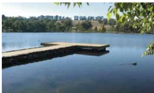
RIGHT Jetty, Macquarie River, Cabonne LGA
