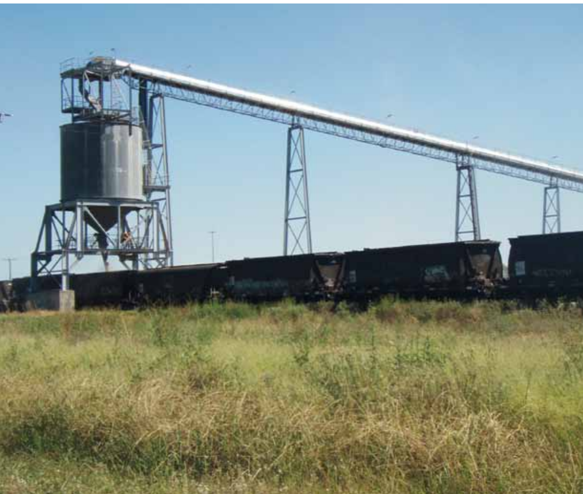
BELOW Loading the grain trains in Trangie
